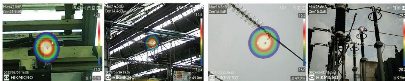
Gas Leak Detection
