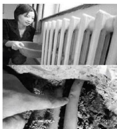
Heating Pipes/ Underfloor Heating Pipe Leaks
