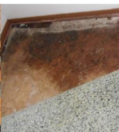
Leak Under The Floor
