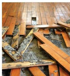
Leak Under The Floor
